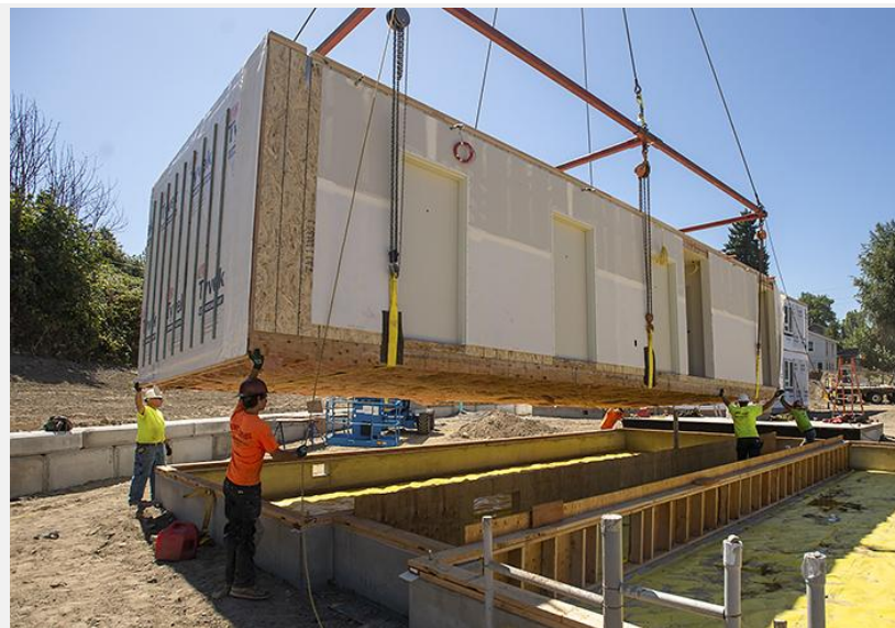
Cody Humphrey, foreground, and Pete Victoor, director of operations for Mods PDX, help guide a modular unit into place atop a foundation. (Josh Kulla/DJC)
