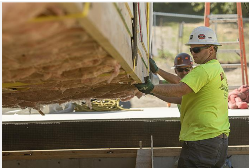
Cody Humphrey helps guide a modular unit into place. (Josh Kulla/DJC)
