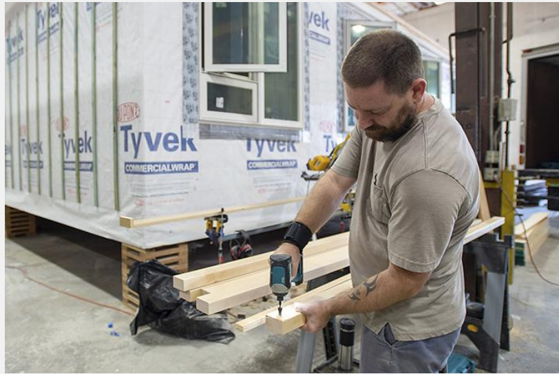
Carpenter Ben Jenkinson of Rockwood Cabinetry prepares strips of interior trim at the Mods PDX warehouse in North Portland. (Josh Kulla/DJC)
