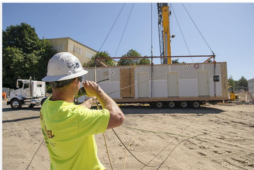
Cody Humphrey talks to a crane operator as he helps guide a modular unit into place. (Josh Kulla/DJC)
